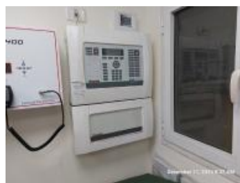
Smoke detection control board.jpg
