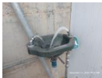
Test of eye-wash station.jpg
