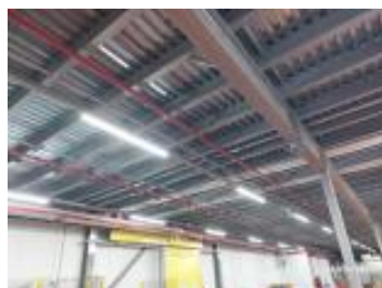
Sprinkler system pipelines.jpg
