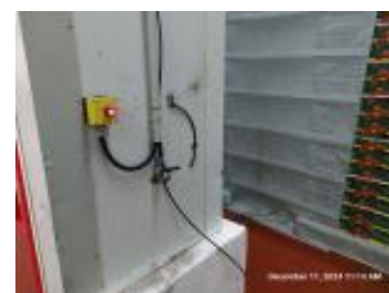
Emergency button in the cooling room.jpg
