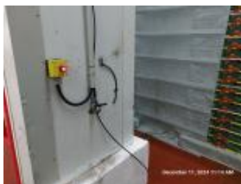
Emergency button in the cooling room.jpg
