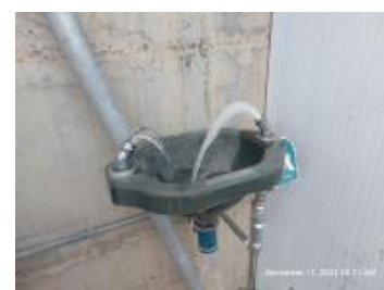
Test of eye-wash station.jpg
