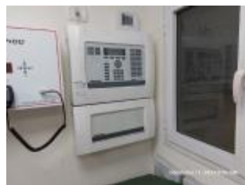
Smoke detection control board.jpg
