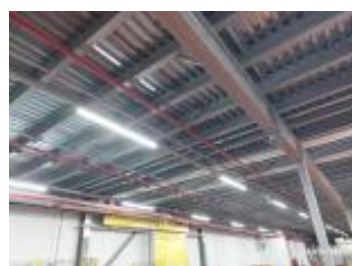
Sprinkler system pipelines.jpg
