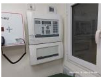
Smoke detection control board.jpg
