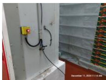
Emergency button in the cooling room.jpg
