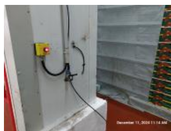
Emergency button in the cooling room.jpg
