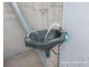
Test of eye-wash station.jpg
