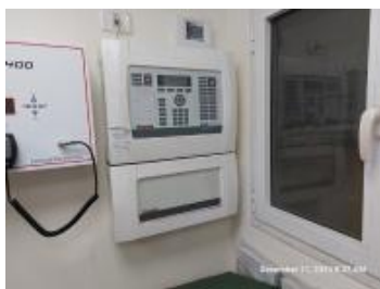
Smoke detection control board.jpg
